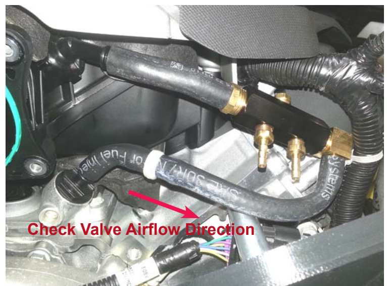
Vacuum Manifold Installed
